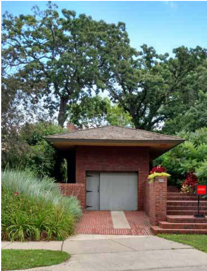
The only really visible part of the Willey house designed by Wright, viewed from Bedford Ave SE. Thick vegetation plus a security warning sign preclude any good photos of the rest of the structure--lots has grown up around it in 80 years.
